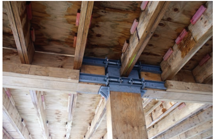
Figure 10 Face fixed 'plug and play' connectors to primary beams
