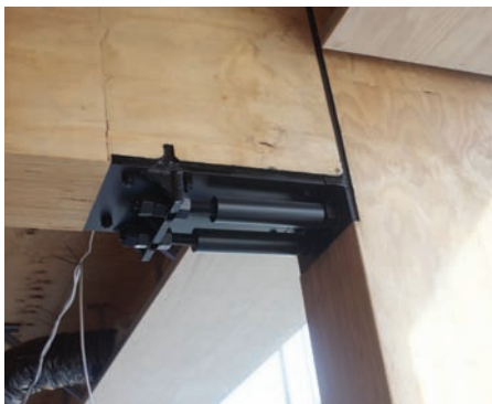
Figure 7 'Plug and play' connector energy dissipaters
