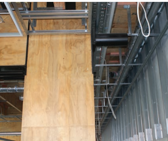
Figure 7 'Plug and play' connector energy dissipaters
