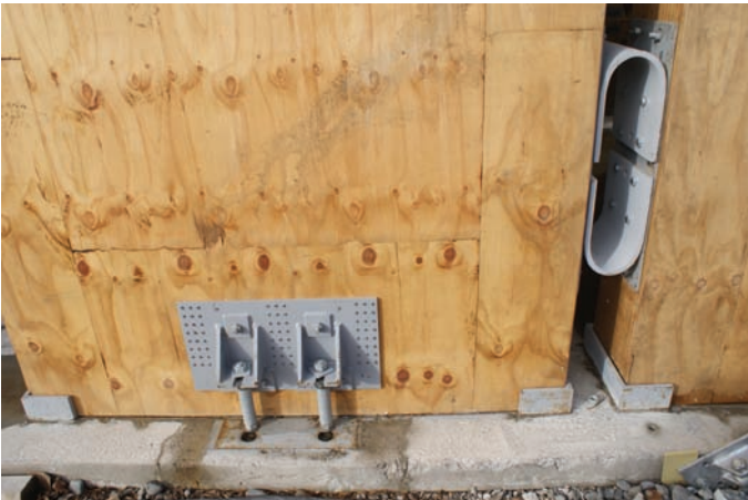
Figure 9 Two types of energy dissipater at base of shear walls
