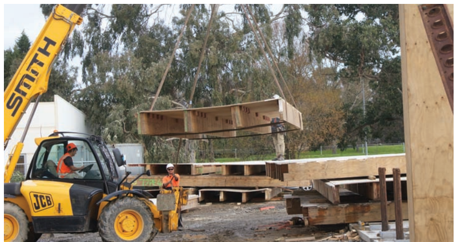
Figure 11 Pre-fabricated timber concrete composite floor units
